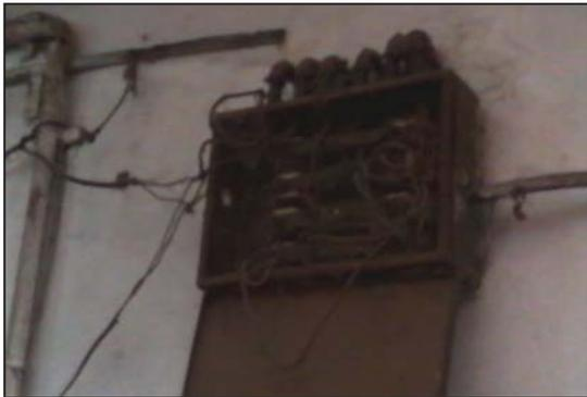
Photo 3: Electrical switches boards are open and prone to hazard. Short circuits are the major source of fire in hospitals in India.
